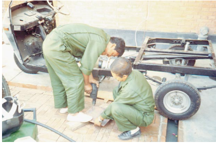
Choudry and Ram drill brackets.
